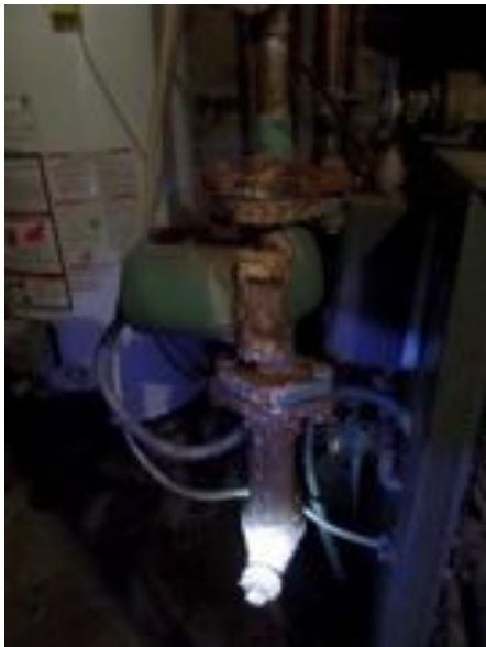
Rust/Corrosion
