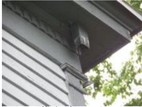
Missing downspout
