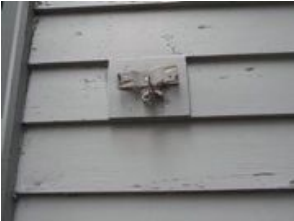
Missing fixture
